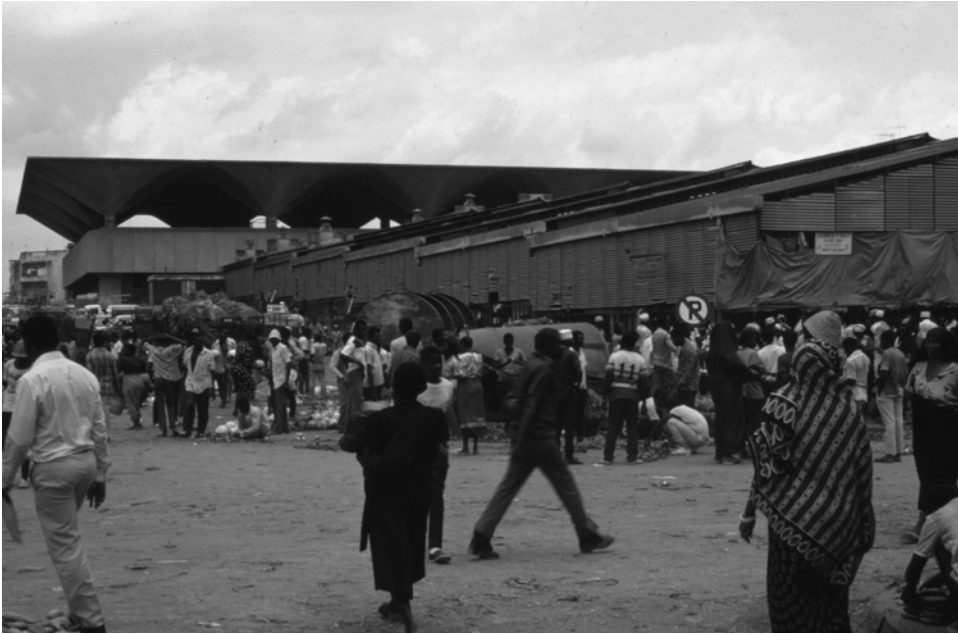
Figure 2.6 Kariakoo market building, Dar es Salaam, housing the city's main wholesale market.
