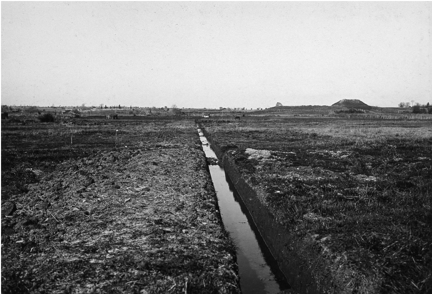
FIGURE 4.2 Nettuno, Italy: a long, narrow drain (to aid mosquito control) in a field. Photograph, ca. 1910–1940.
